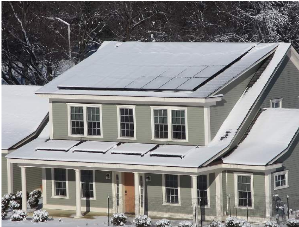
Net-Zero Energy Residential Test Facility (NZERTF) in the snow (14531301000).jpg, Credit: NIST – National Institute of Standards and Technology
